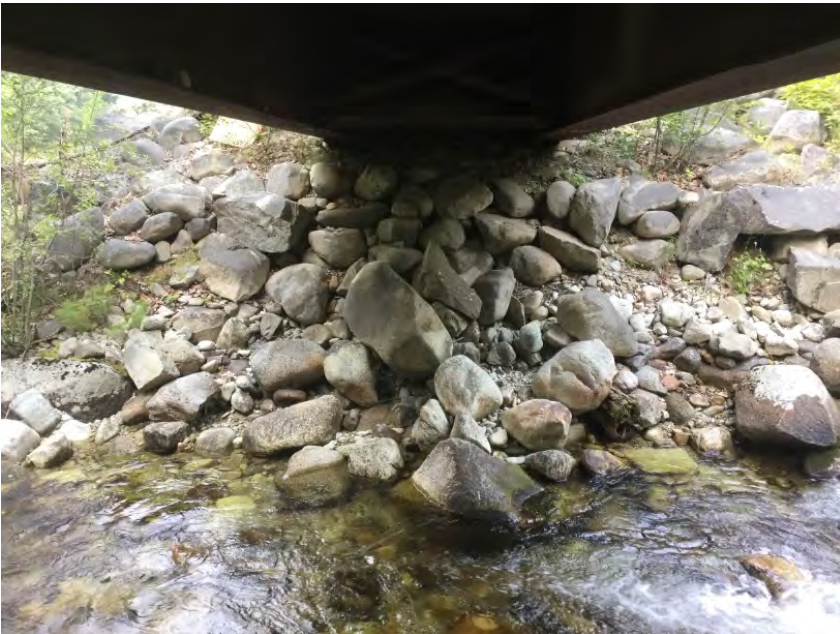
Right Bank Abutment when facing downstream
