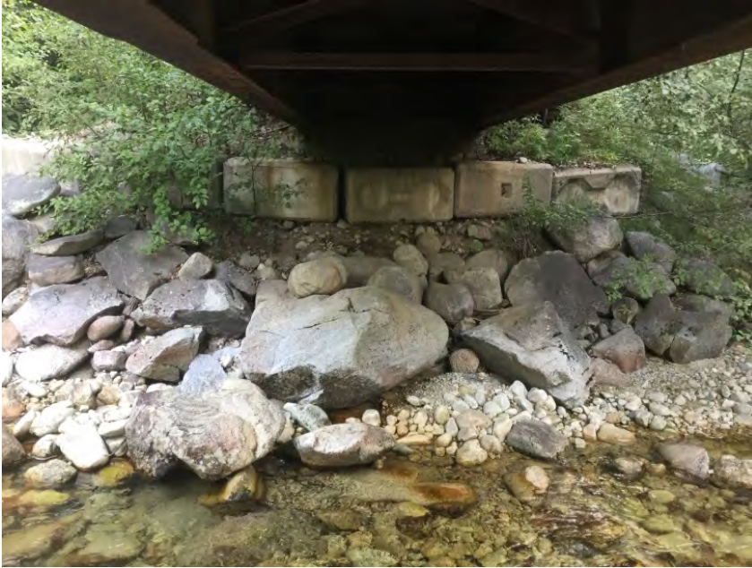
Left Bank Abutment when facing downstream
